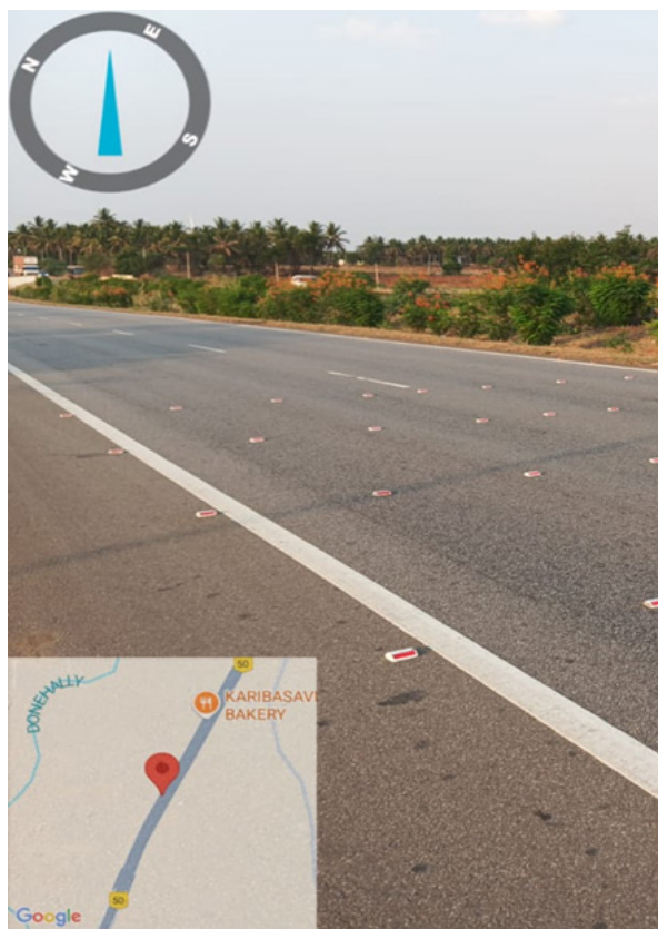
Reflective Raised Pavement Markers for improving visibility and speed calming at Hampi expressway
